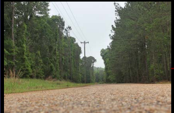
View of Paved Road Frontage
