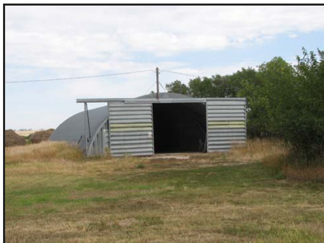
40'X70' Steel Quonset
