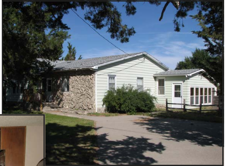
Remodeled house with Sunroom Addition
