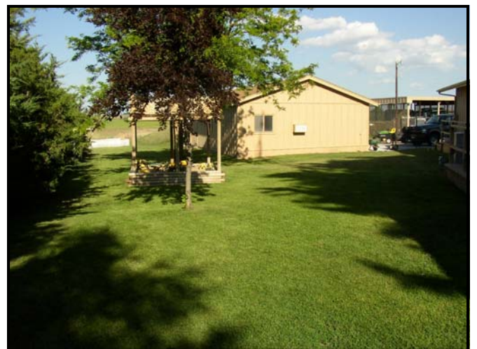
Office in unattached garage & RV carport in back
