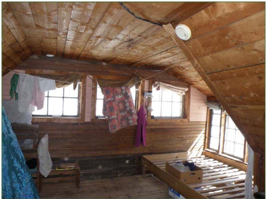
Second floor sleeping quarters.
