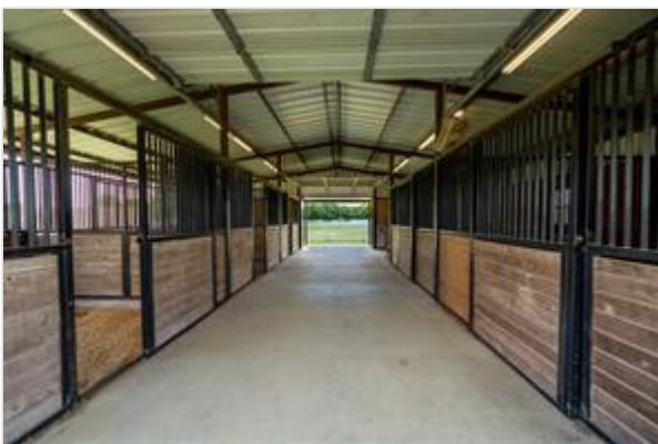
BARN 2 INTERIOR...Concrete Center Aisle, 3 Stalls On Left Side Of Photo And 2 Stalls Plus Storage Area On Right Side Of Photo
