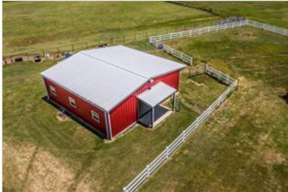
BARN 2 EXTERIOR...36X36 With Five 12x12 Stalls
