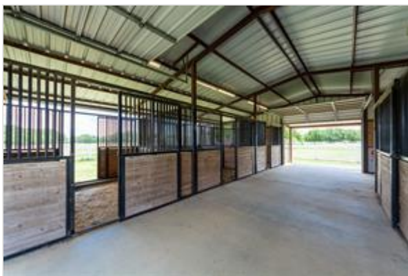
BARN 2 INTERIOR...Extra Photo, The Three 12x12 Stalls On Left Side Of Photo Each Have An Exterior Sliding Stall Door To The Outside
